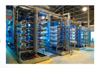
pores under pressure to remove the floc formed during coagulation including organic colour and solids as well as any microscopic organisms including bacteria, Cryptosporidium and Giardia. This also removes the coagulant chemicals which are bound up within the floc. Each filter train is backwashed approximately every 40 minutes of operation time and is chemically cleaned every 24 backwashes. The backwash waste water is collected and treated in the wastewater treatment system.
