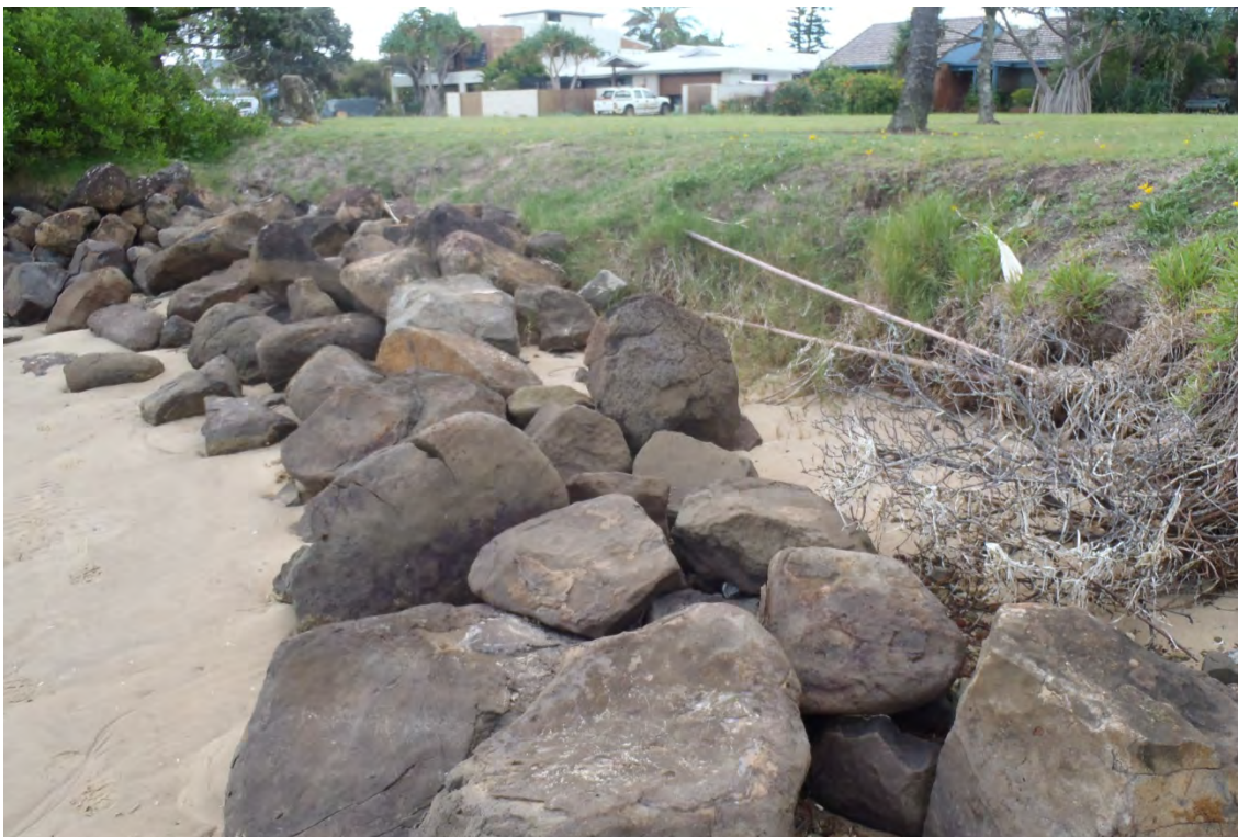
Figure 3: East Arm erosion showing rock wall to be reinstated
