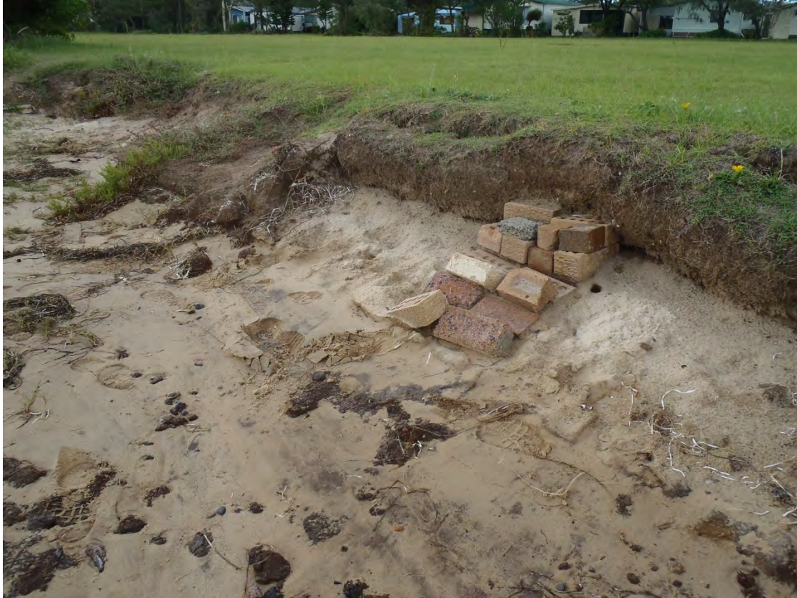
Figure 4: East Arm erosion with poor waterway access to be regraded to beach
