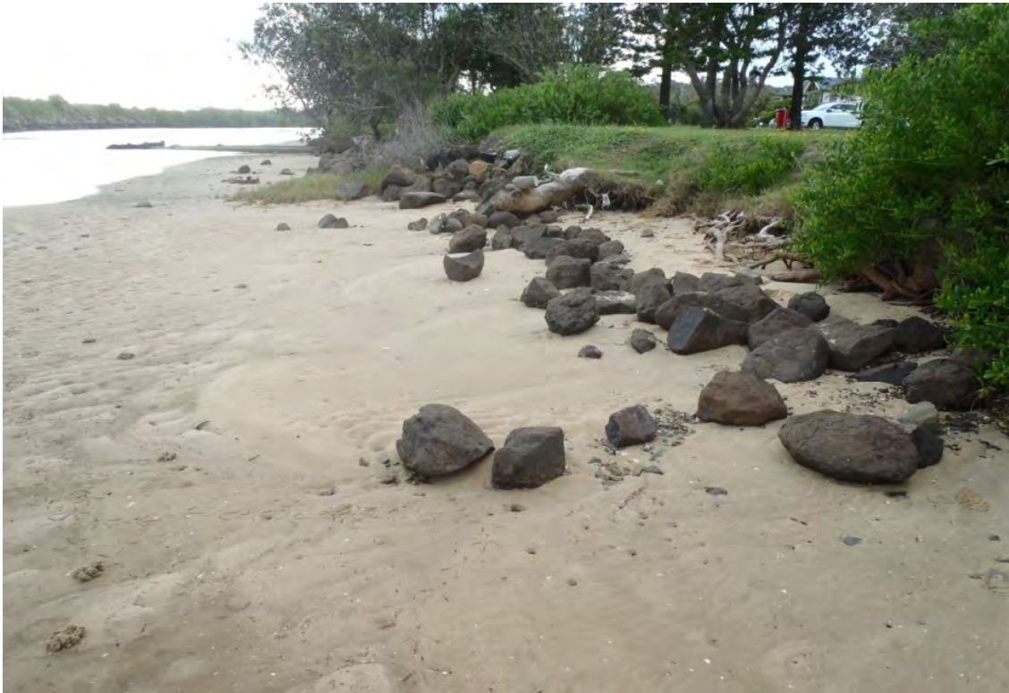
Figure 2: East Arm erosion and failed erosion control - location of proposed rock revetment wall
