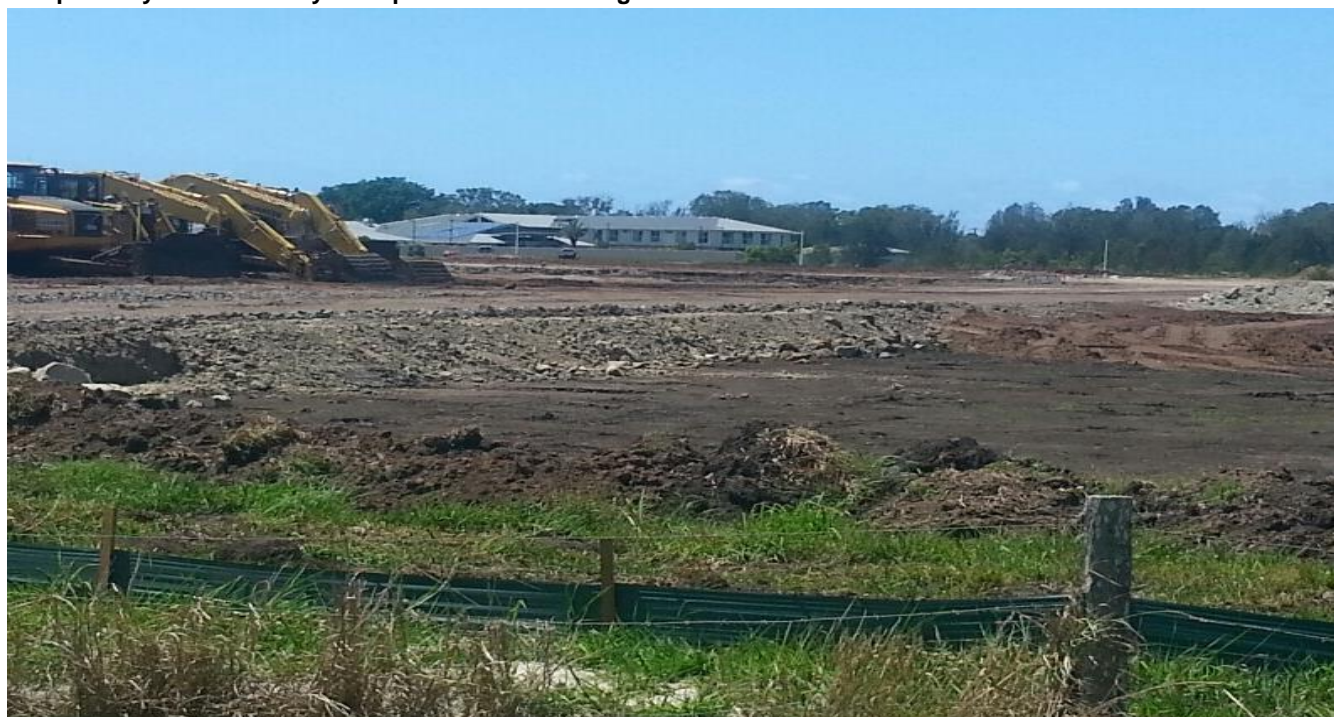
Photograph 11 – Broad-acre filling, Corkys Lane, Ballina. Filling on this scale generally does not create adjoining land compatibility issues as may be experienced with filling on infill sites.
