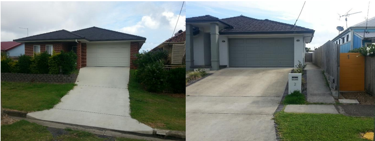
Photograph 6 and 7 – Examples of dwellings in Ballina built using slab on ground construction after significant site filling.
