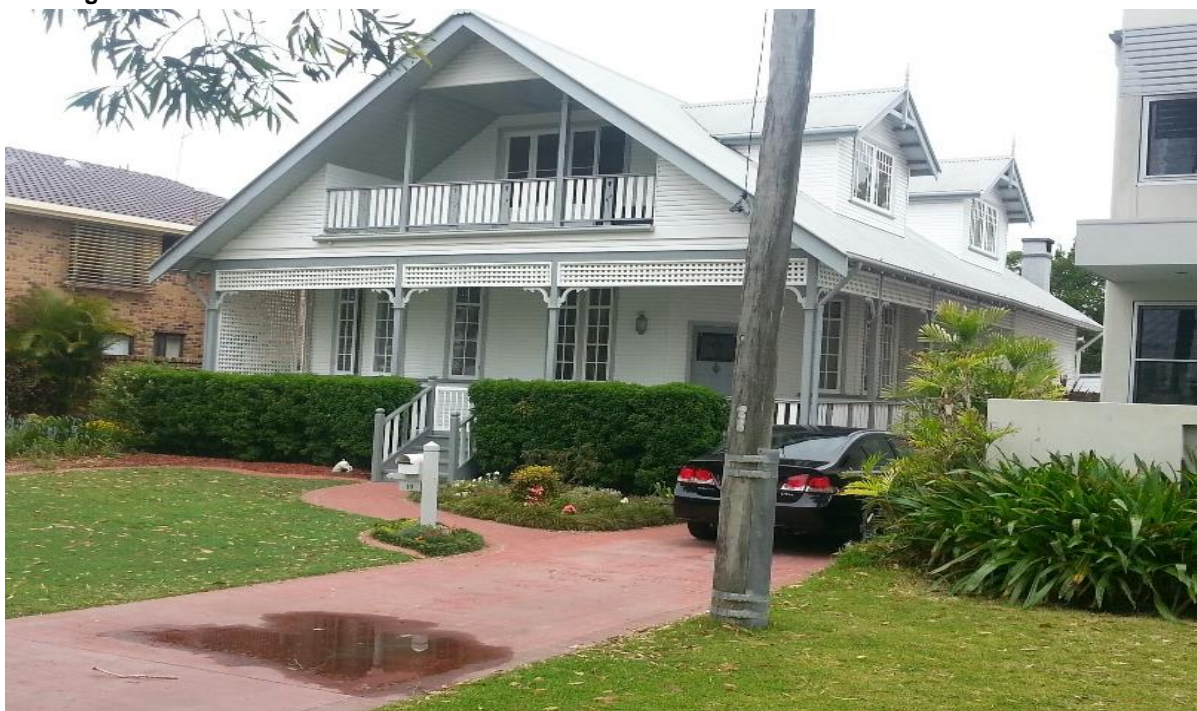
Photograph 13 – Renovated dwelling Fox Street, Ballina, Design more resilient to climate change. Use of pier and beam footing construction, lightweight materials, balcony under main roof and use of a light colour palette typifies elements of the suggested Ballina Style. Bedrooms under gable roof, and use of dormers, effective in reducing height impacts and creating character.
