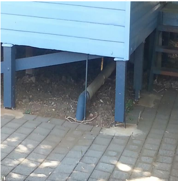
Photograph 15 & 16 – Piers used to support residential building on Ballina Island. In one case a restumped dwelling and in the other a new secondary dwelling on galvanised steel piers.
