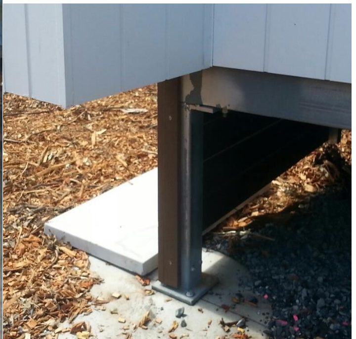
Photograph 15 & 16 – Piers used to support residential building on Ballina Island. In one case a restumped dwelling and in the other a new secondary dwelling on galvanised steel piers.
