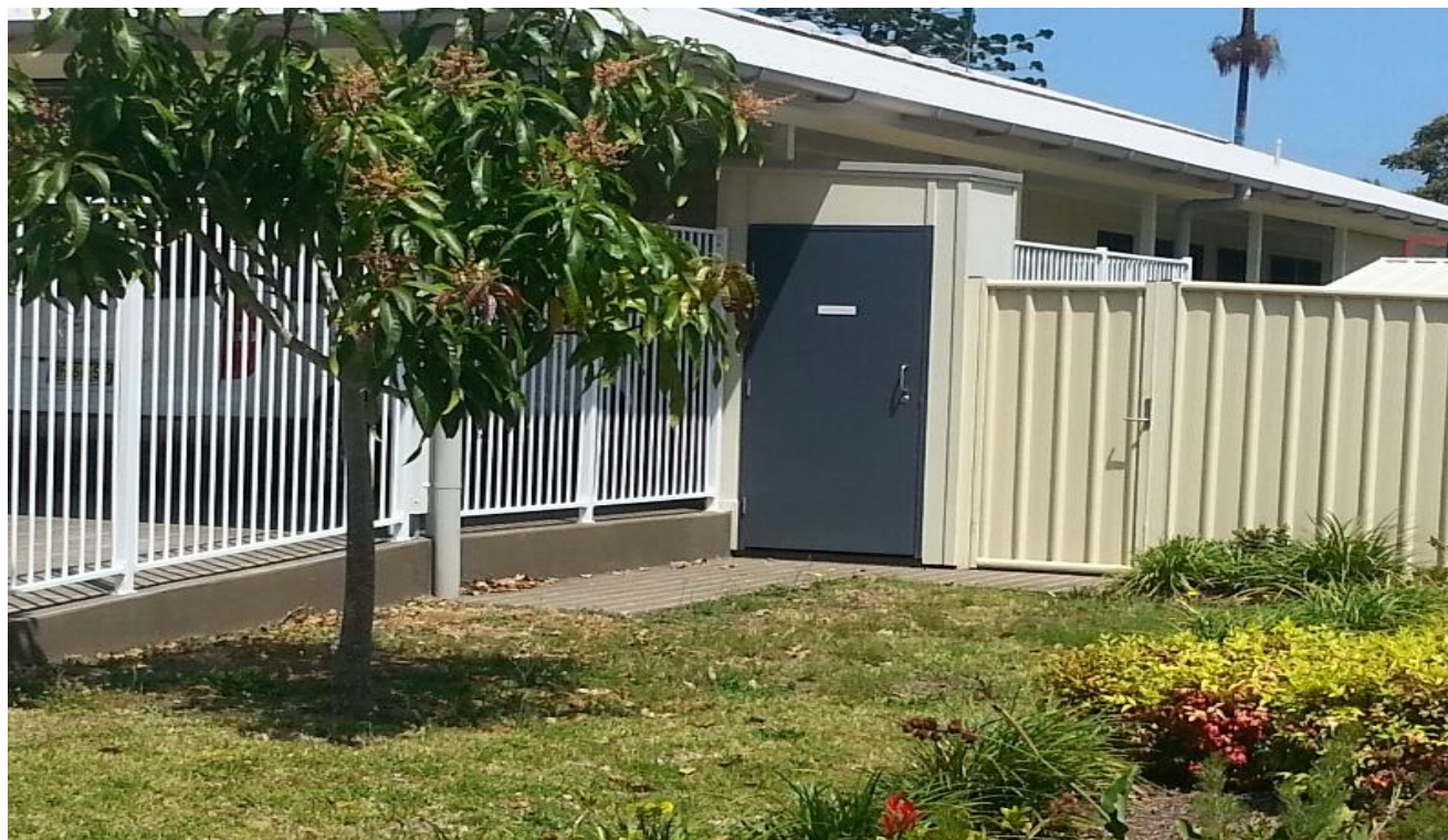
Photograph 10 – Department of Commerce, 2008 Group Home Development, Burnet Street Ballina, Side View showing Raised Slab and Existing Site Levels.
