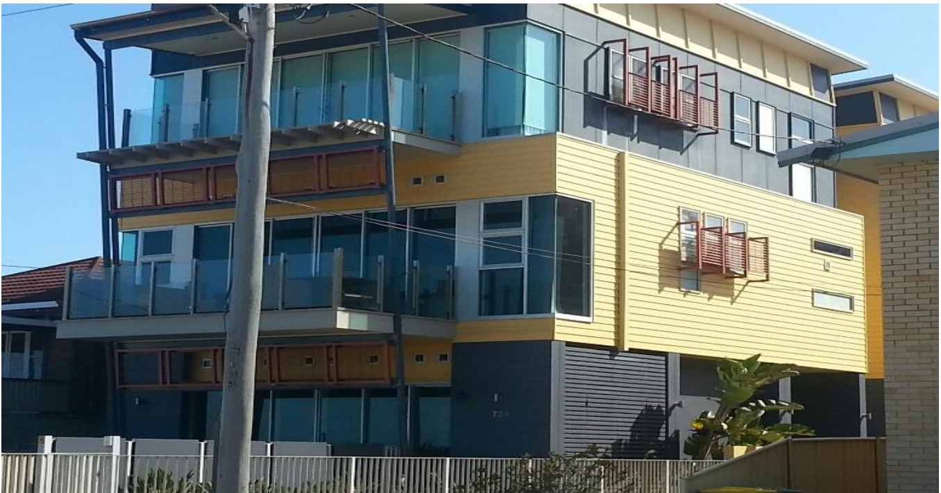
Photograph 19 – A residential flat building located in Currumbin, Queensland which has incorporated light-weight materials within external walls.
