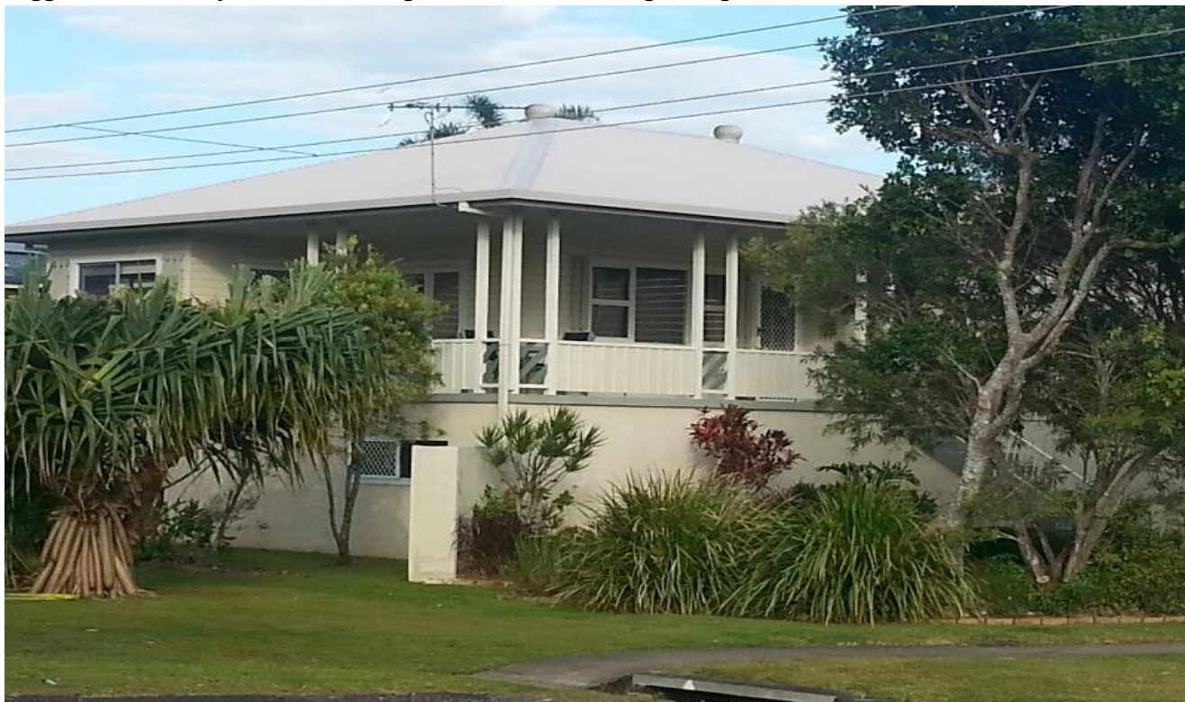
Photograph 12 – Renovated dwelling Tamar Street, Ballina, Design more resilient to climate change and is typical of the suggested Ballina Style with main living areas on first floor. Light-weight materials also used on first floor.
