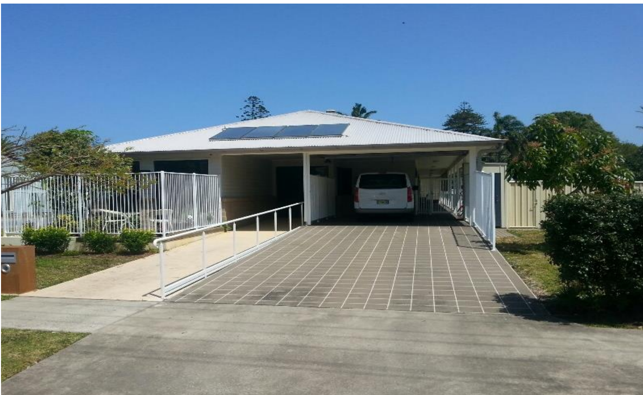
Photograph 9 – Department of Commerce, 2008 group home development, Burnet Street Ballina. Dwelling raised with existing site levels retained for yard areas. Construction costs reduced through elimination of whole of site filling. Development also more compatible with adjoining development.
