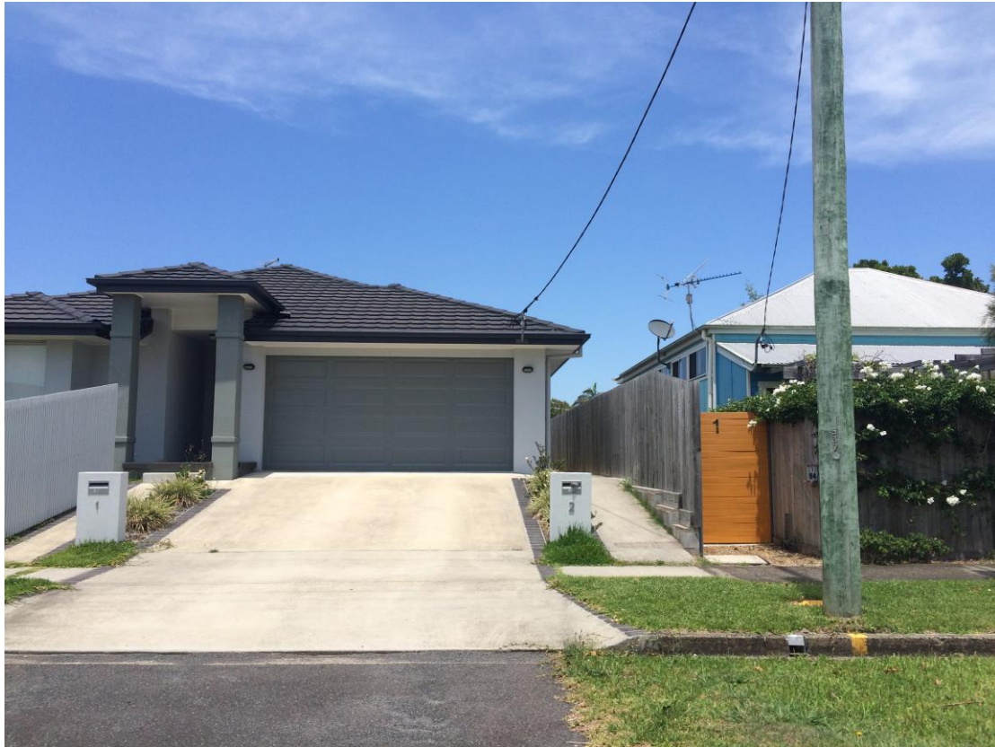
Figure 7 New “filled” lot interrupting natural levels of ground height
