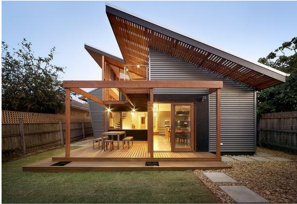
Photo – Example of Ballina style features within this dwelling (internet photo) include striking modern skillion roof design, lightweight materials for walls and roof, dwelling on piers not slab on ground. Ground floor deck should be covered to qualify as a Ballina style component.
