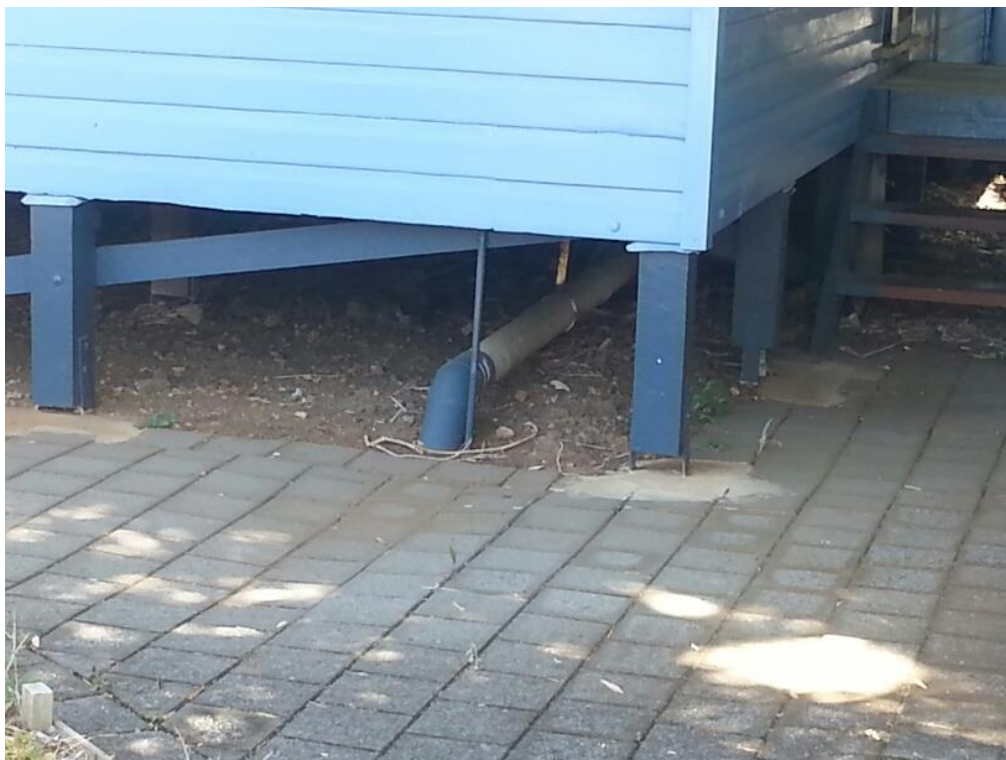
Ballina style foundation elements. This photo shows foundations contained within a building originally built as a dwelling house now used for commercial purposes. Services are readily accessible, in this case stormwater, which facilitates easy disconnection should need to raise building arise.
