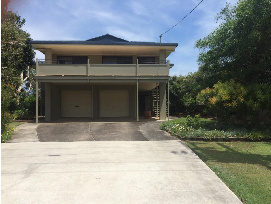
Figure 10 A renovated house that has elements of Ballina style - elevated floor, long eaves. Although predominantly built out of masonry and heavyweight construction it connects to Ballina style with some design features.
