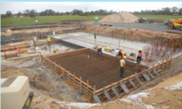
Ballina Wastewater Treatment Plant Upgrade - steel reinforcement being placed in the formwork for the base slabs to the membrane bio-reactor tank.
