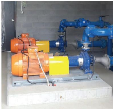
Pump station that feeds water to Newrybar from the Knockrow Reservoir. Newrybar is at a higher elevation to the reservoir and requires pumps to deliver water to properties at Newrybar.
