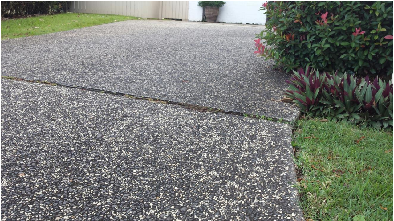
Photo No. 6 – The step in the contraction joint in the driveway slab at the property boundary as photographed on 27 April 2018 did not exhibit any significant change over the past 12 months.
