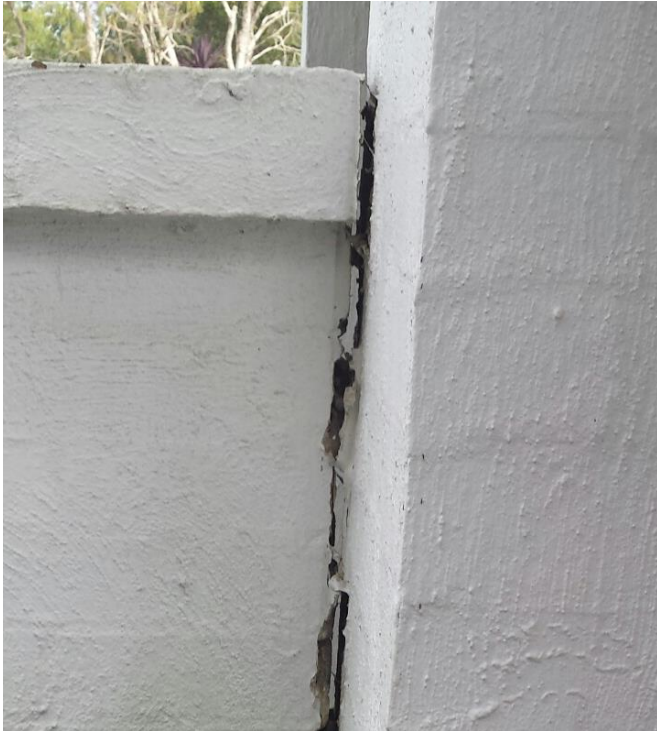
Photo No. 7 – As photographed on 6 April 2017, lifting and rotation of the brick privacy wall on the western side of the garage had opened up a gap in the vertical joint with the house.
