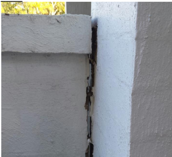
Photo No. 8 –The vertical joint between the brick privacy screen and the house as photographed on 27 April 2017. This joint has widened by about 4mm and the privacy screen has lifted by about 10mm over the past 12 months.
