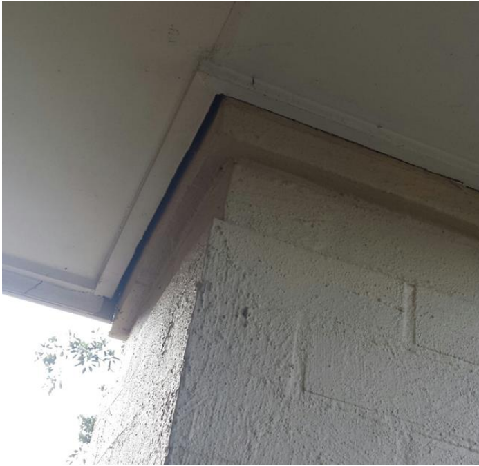
Photo No. 1 – Leaning brick pillar at the entry to the house as photographed on 6 April 2017.
