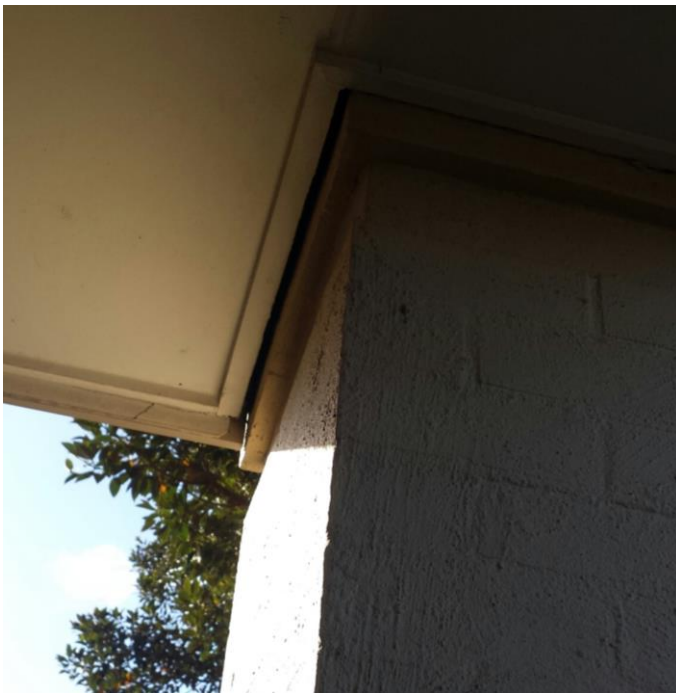
Photo No. 2 – The leaning in the brick pillar at the entry as photographed on 27 April 2018. The lean does not appear to have deteriorated over the past 12 months.
