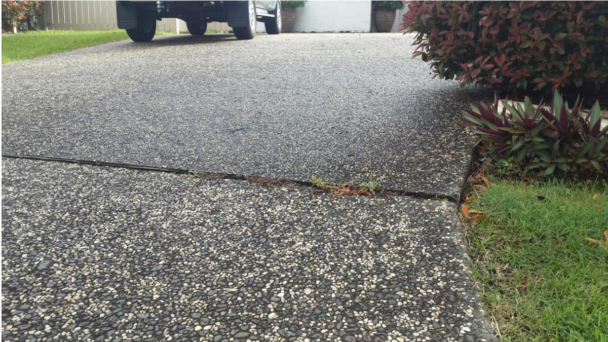
Photo No. 5 – A step in a contraction joint in the driveway slab at the property boundary as photographed on 6 April 2017.
