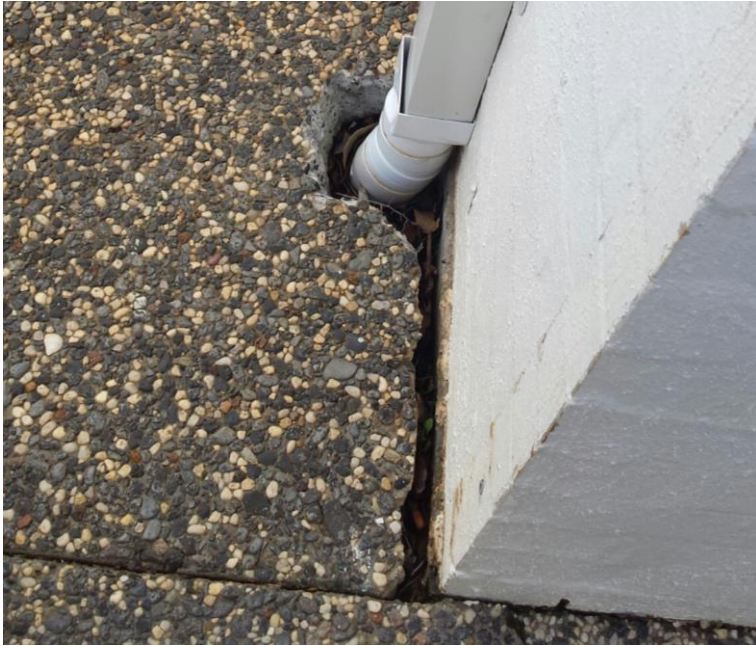
Photo No. 9 – Separation of the 1.3metre wide path from the wall on the western side of the house as photographed on 6 April 2017
