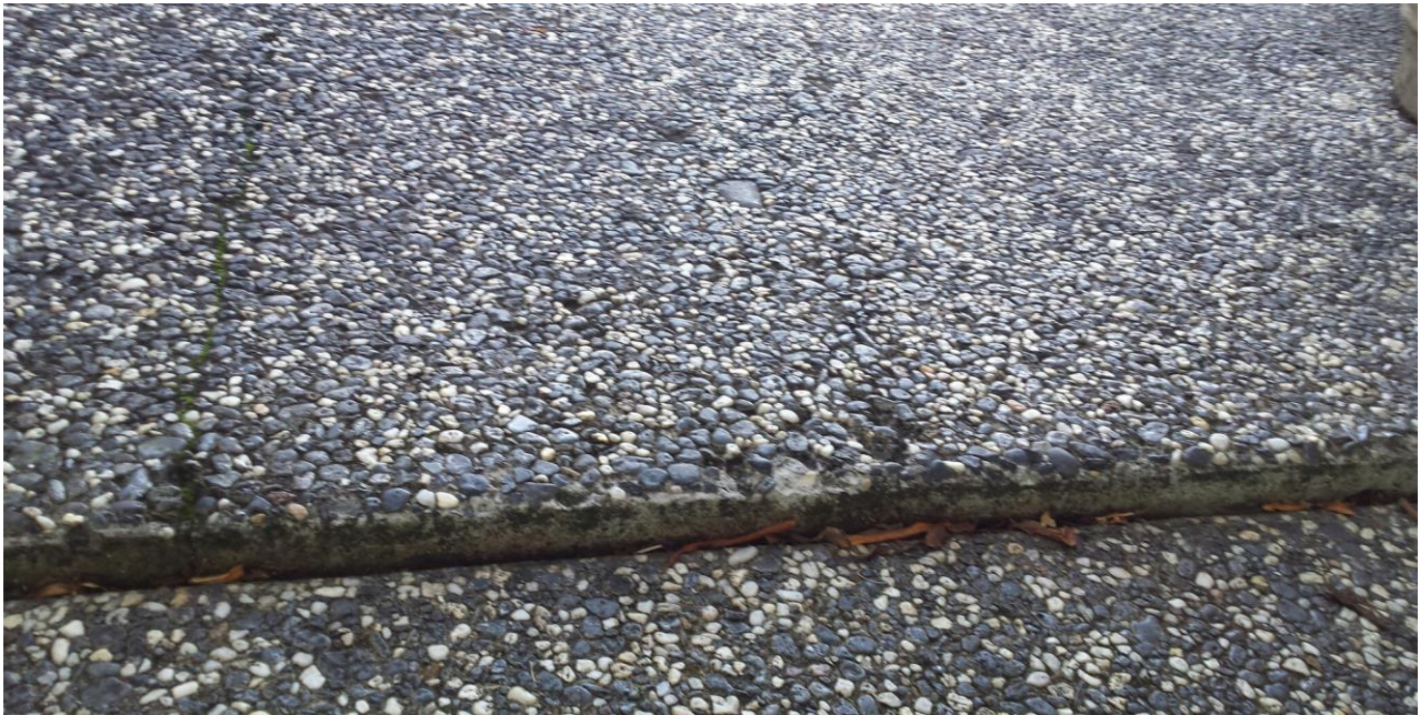
Photo No. 4 – Lifted concrete driveway slab abutting the garage floor slab as photographed on 27 April 2018 when the step at the joint was measured at 35mm high.
