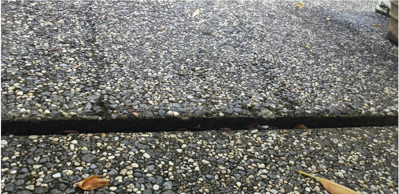
Photo No. 3 – Lifted concrete driveway slab abutting the garage floor slab as photographed on 6 April 2017. At the time the step at the joint was measured at 25mm high.
