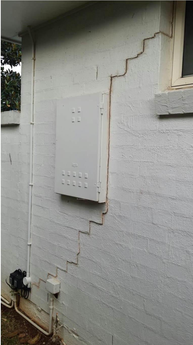
Photo No. 12 – Cracking in the brick wall at the south-eastern corner of the house as photographed on 27 April 2018. This crack does not appear to have deteriorated over the past 12 months.
