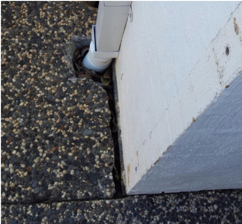
Photo No. 10 – Separation of the 1.3metre wide path from the wall on the western side of the house as photographed on 27 April 2018. The does not appear to have been any significant change since April 2017.
