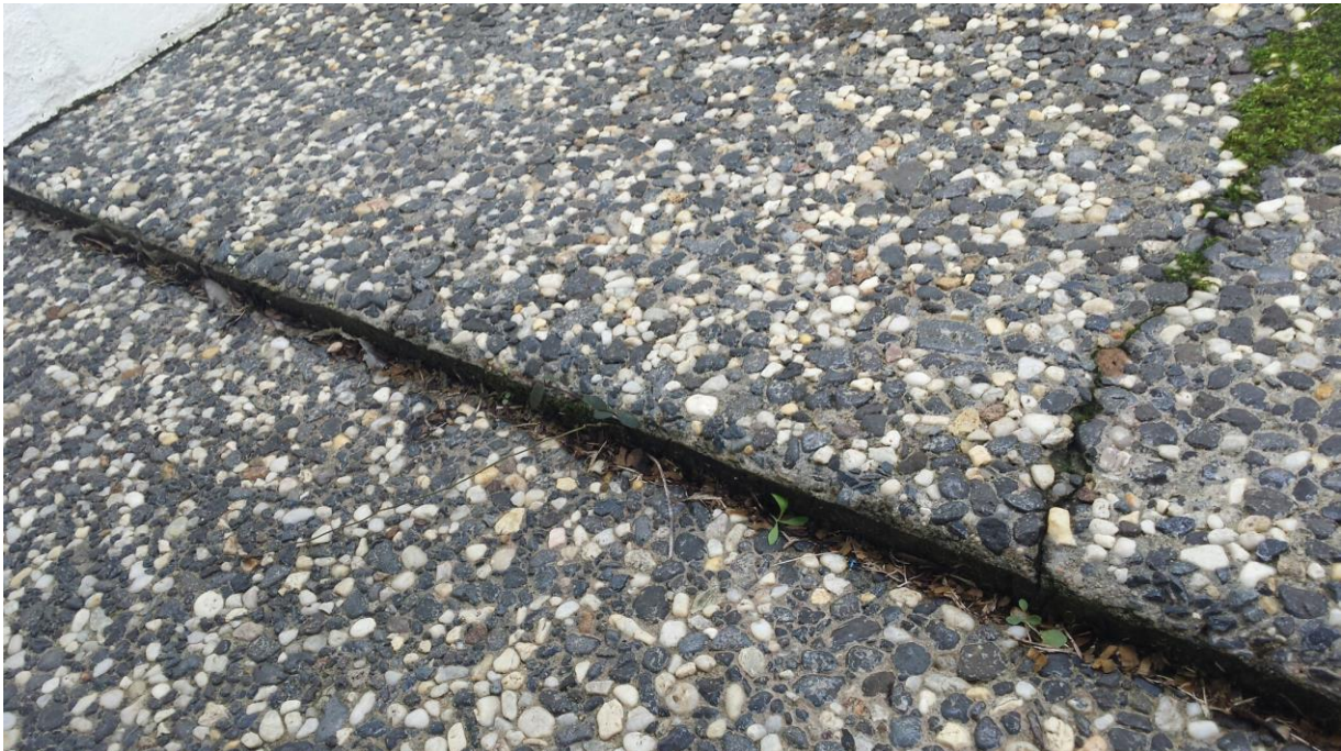
Photo No. 6 – A step and crack in the slab behind the privacy screen on the western side of the garage.
