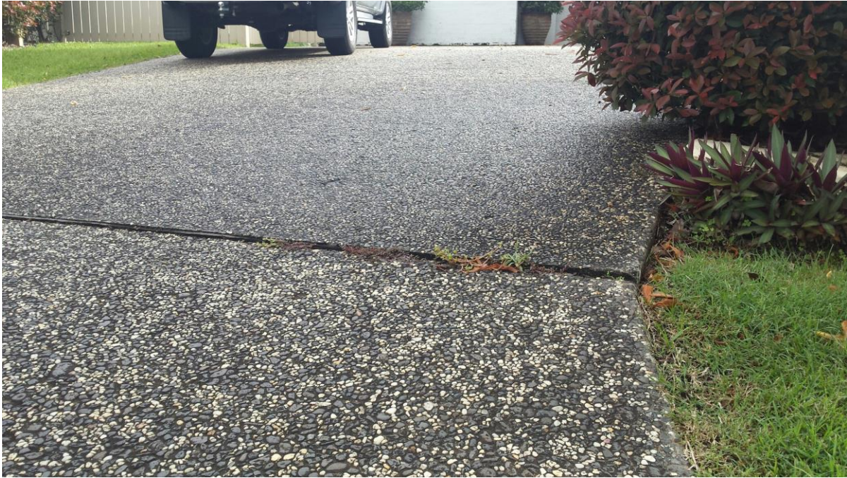
Photo No. 5 – A step in a contraction joint in the driveway slab at the property boundary.
