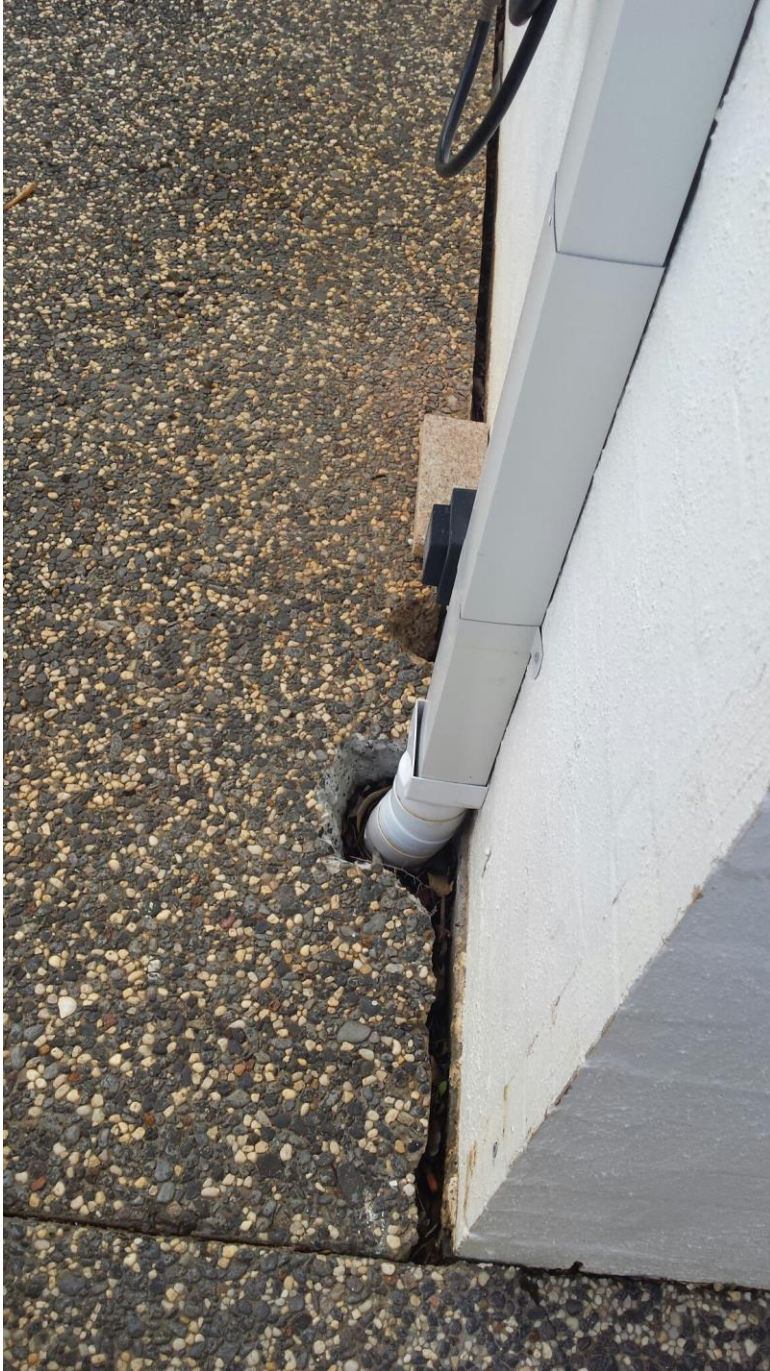
Photo No. 8 – Separation of the 1.3metre wide path from the wall on the western side of the house
