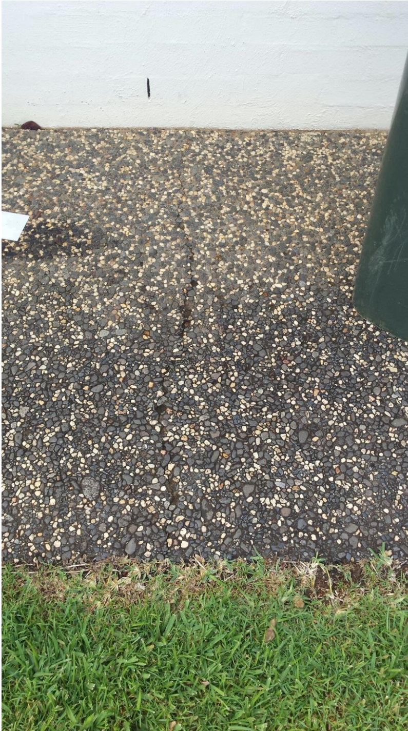
Photo No. 9 –A crack in the 1.3 metre wide concrete path on the western side of the house
