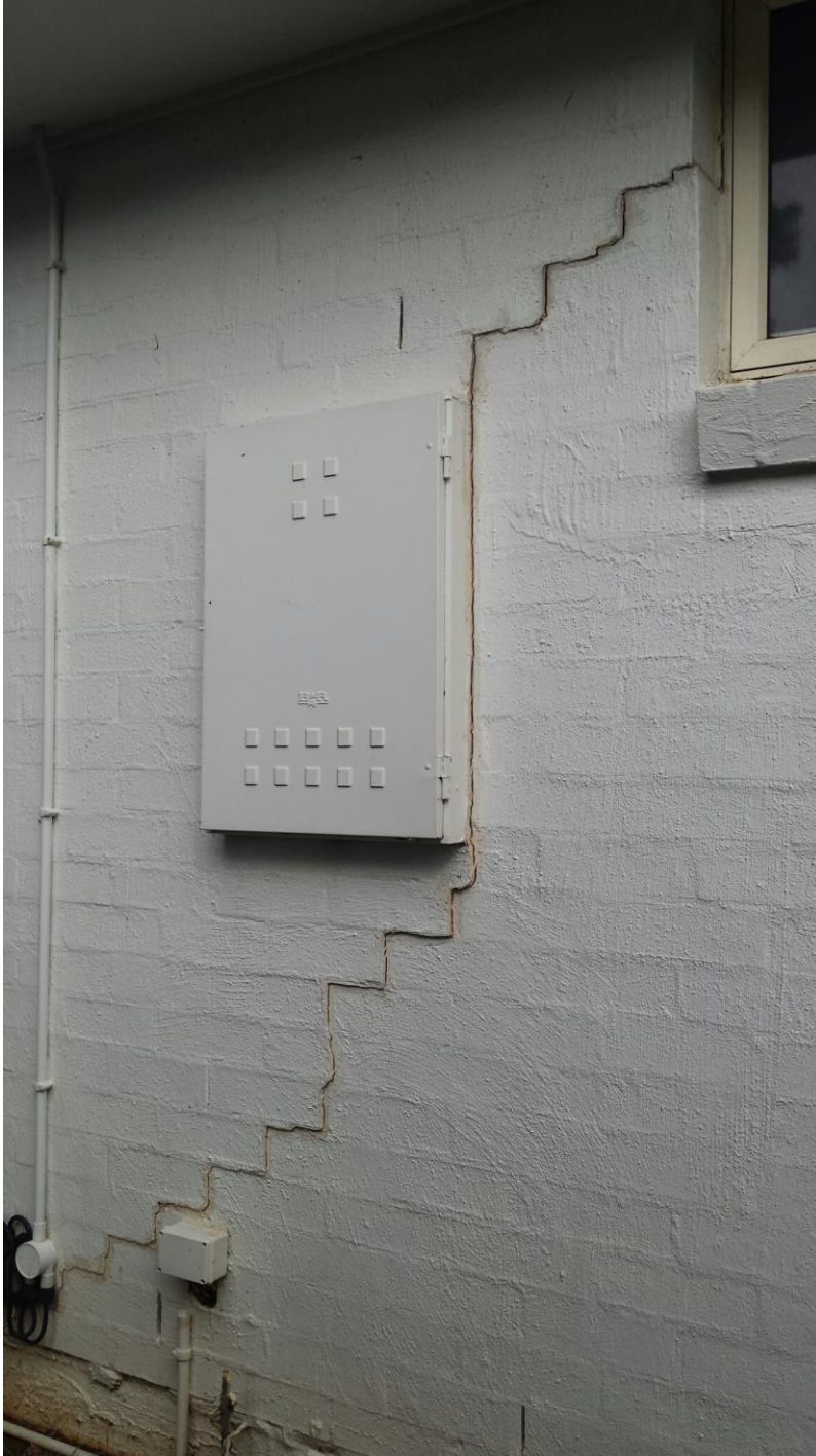
Photo No. 10 – Cracking in the brick wall at the south-eastern corner of the house.
