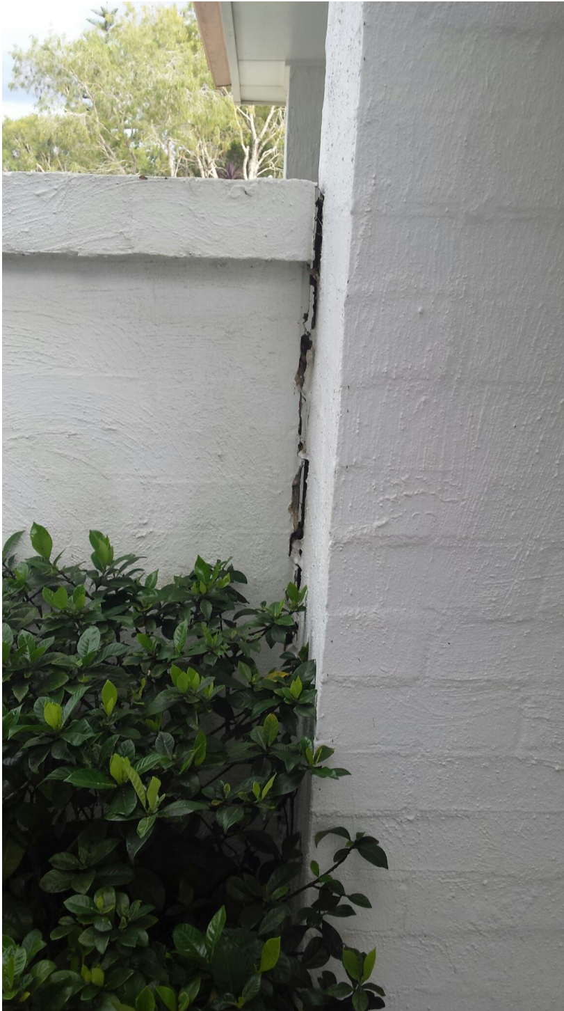
Photo No. 7 – Rotation of the brick privacy wall on the western side of the garage as evident from the gap that has opened up in the vertical joint.
