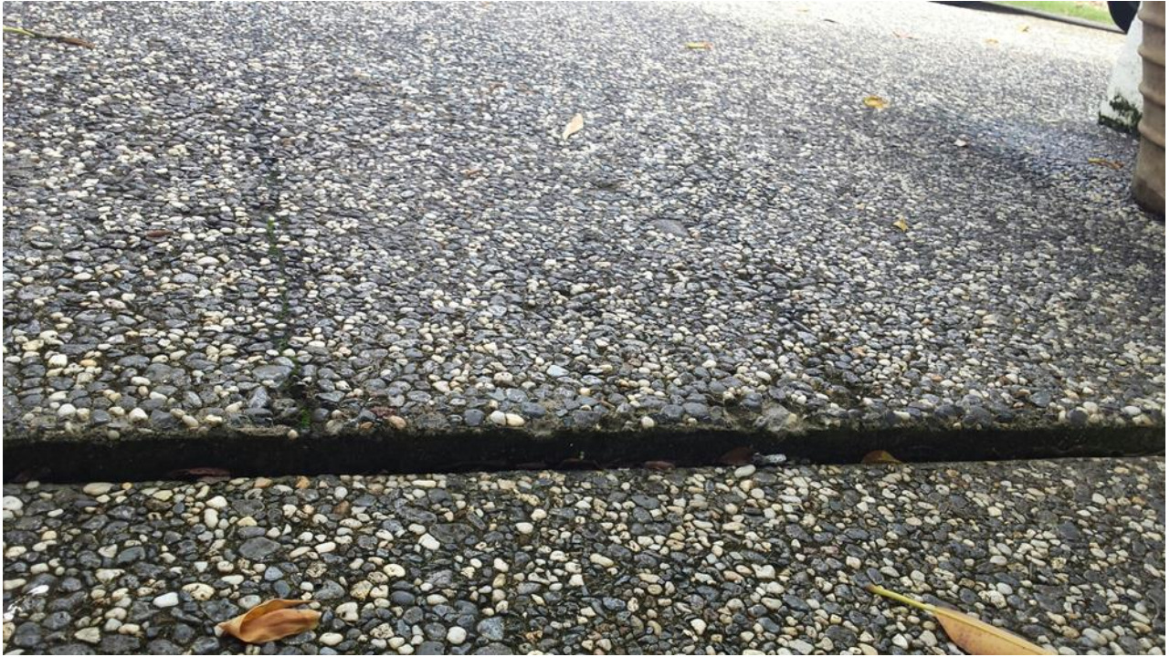
Photo No. 3 – Lifted concrete driveway slab abutting the garage floor slab. Note the presence of cracks.
