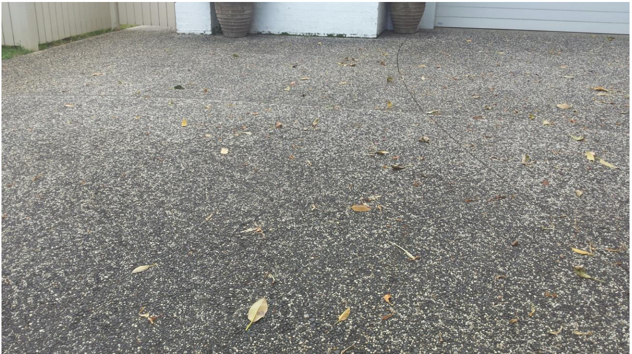
Photo No. 4 – Reflected cracking across a joint in the driveway slab.
