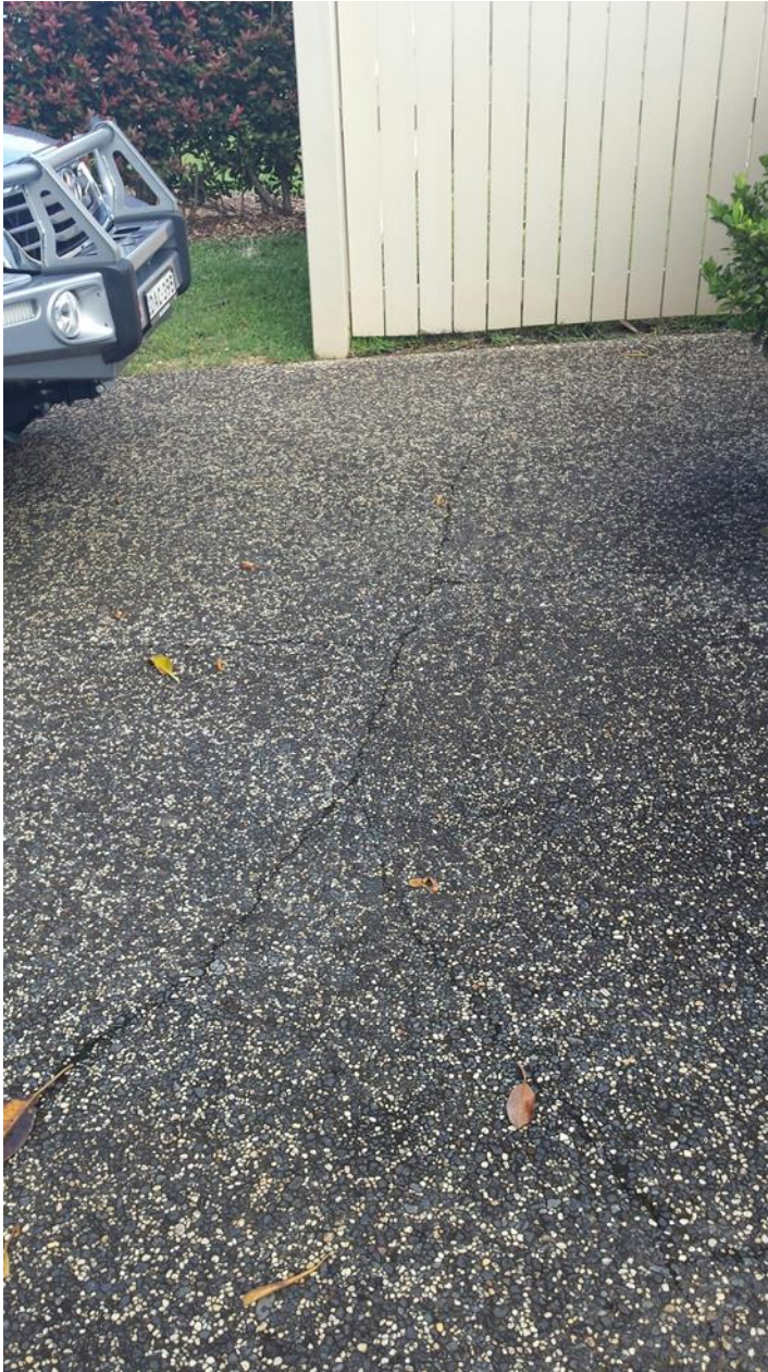
Photo No. 2 – Typical cracking of the concrete driveway slab abutting the garage floor slab.
