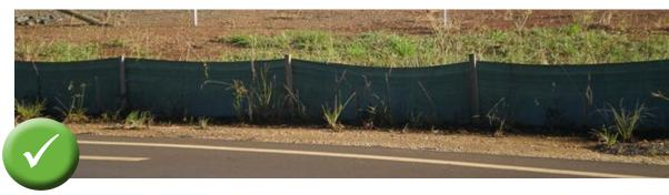
All sediment and erosion controls should be checked at least once each week and after each rainfall event to ensure they are working correctly and identify required maintenance.
