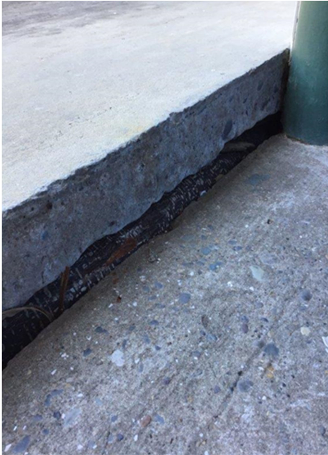
Fig root visible 19m from tree. B. Branch 10/09/2019
