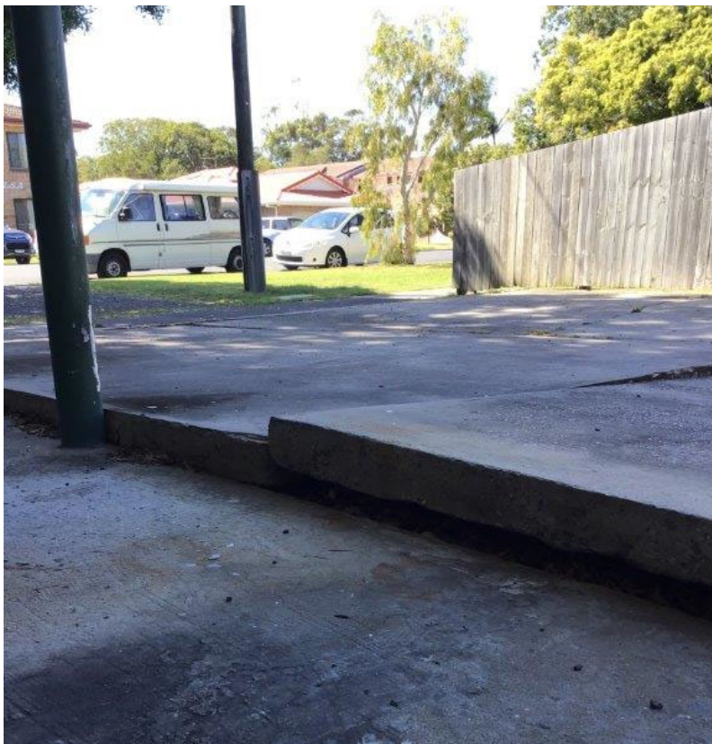
Carpark slabs lifted 150mm by visible root. B. Branch 10/09/2019
