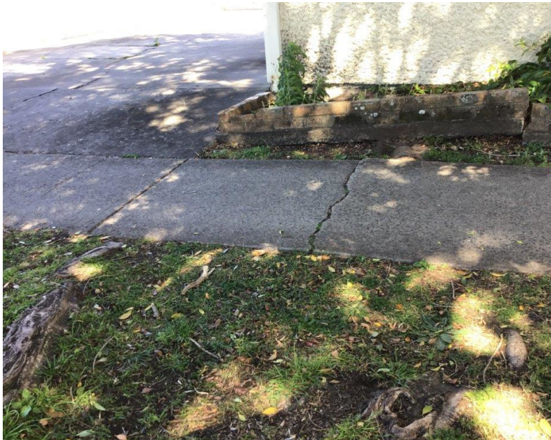
Fig Root heading under footpath on northern side of building. B. Branch 10/09/2019
